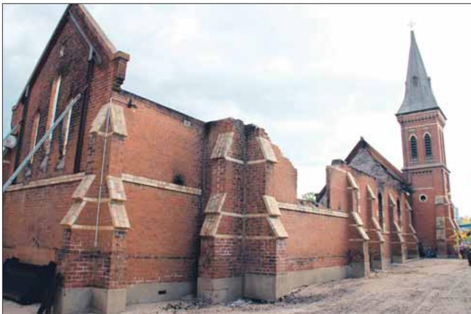
**OPEN HOUSE:** While the fire damaged all the structural timber, which had to be removed, the bell tower is undamaged and it is still hoped some of the brick walls can be retained.
